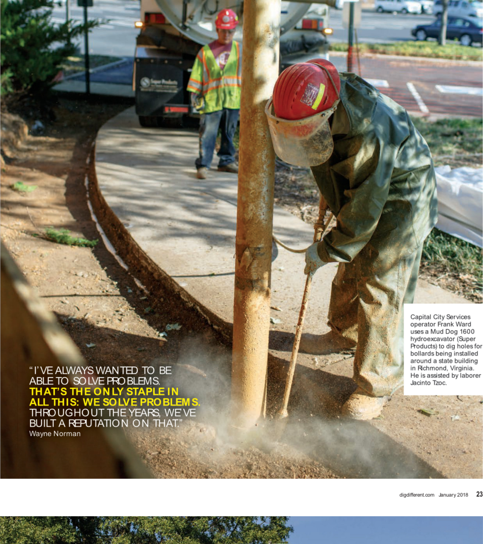
Capital City Services operator Frank Ward uses a Mud Dog 1600 hydroexcavator (Super Products) to dig holes for bollards being installed around a state building in Richmond, Virginia. He is assisted by laborer Jacinto Tzoc.
